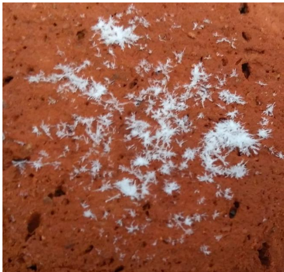
(a) Long needle-shaped salt crystal efflorescence
