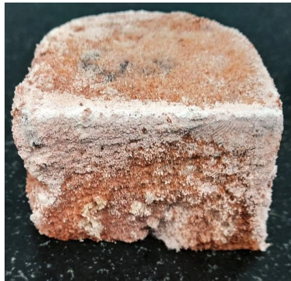
(b) Dense white powdery efflorescence
